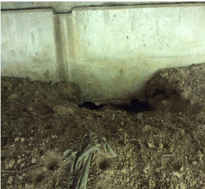
PHOTO 1 Description Abutment 2 right side has 3 large animal holes.
